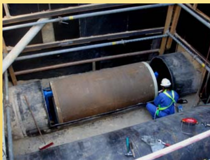
Segment positioned on installation trolley
