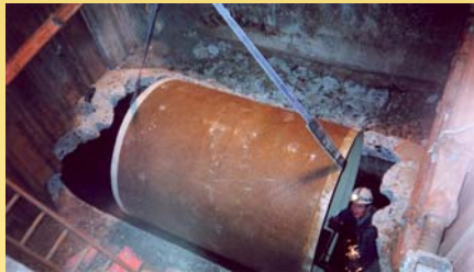
Liner segments in position in pipe invert
