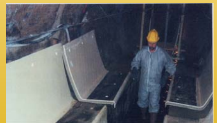
Multipiece Channeline Sections being installed in large, complex shaped sewer
