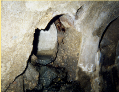
Lateral before rehabilitation
