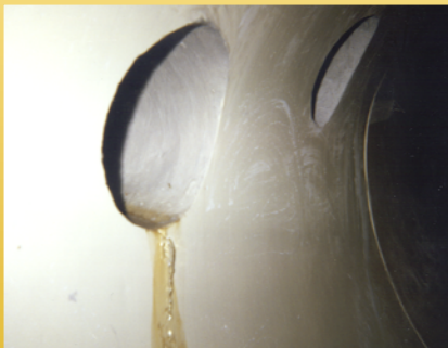
Lateral after rehabilitation
