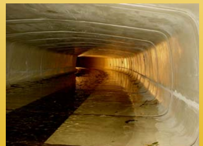
Flattened Box Section
