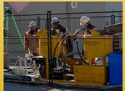
Grout rig for mixing and pumping
