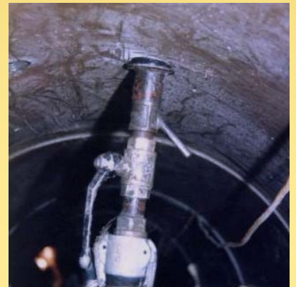
Injection of grout into the annular gap
