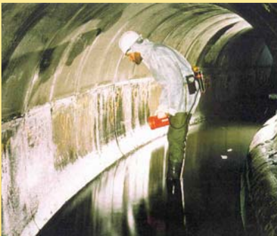
Inspection of Channeline after many Years of service
