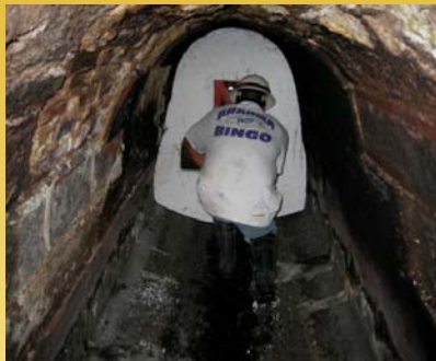
Liner fit being checked with template
