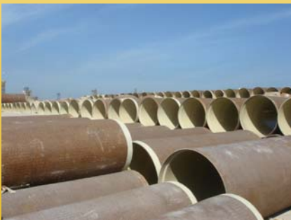
Channeline segments delivered to site Awaiting installation.
