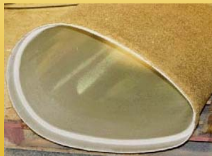
End of Channeline Egg-Shaped Panel Showing Socket Joint
